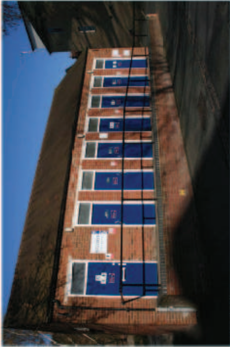
WEST ELEVATION MAIN ENTRANCE TO TOILET BLOCK
